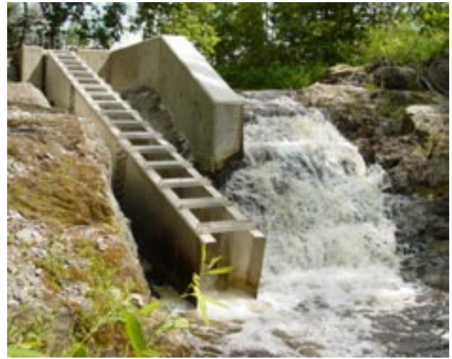
Plymouth Pond Fish Ladder on the Sebasticook River in Plymouth, Maine. Credit: John Catena, NOAA
