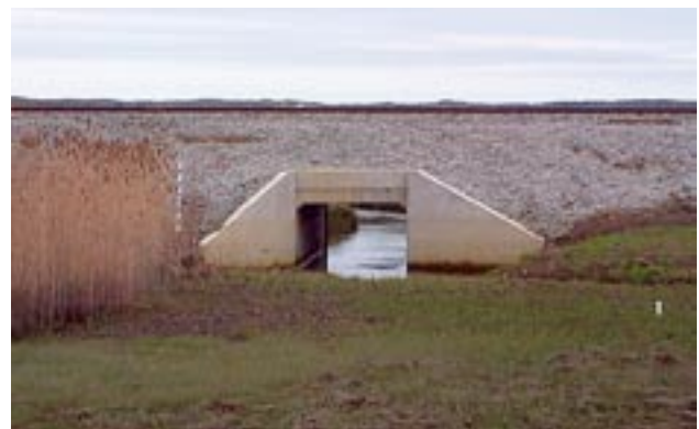
One method of salt marsh restoration is to replace undersized culverts (top) with larger culverts that allow greater tidal exchange (bottom). Top Photo: Massachusetts Wetland Conservation Program; bottom photo: Jon Kachmar
